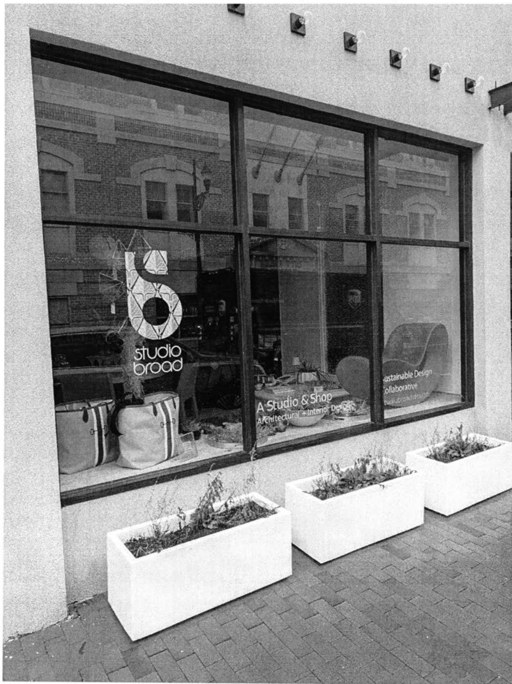
Figure 1 Current Storefront to be modified (Exterior)
