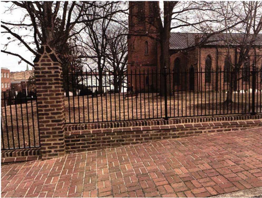
Section of Church Street brick wall base and metal fence that would be modified to receive the new entry for the proposed ADA ramp.
